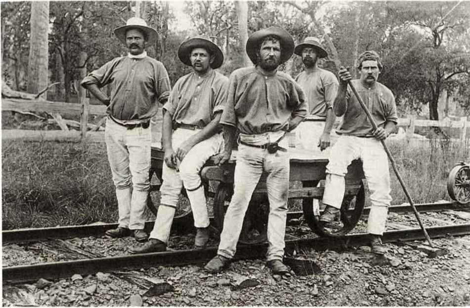
A gang of fettlers on the Ipswich–Toowoomba line in southern Queensland take a tea break. Their moleskin trousers, canvas leggings, flannel tunics and wide-brimmed hats were standard bush labourer's attire. The four-wheeled repair truck on which they sit was used in conjunction with the manually powered trike or trolley, one wheel of which is just visible on the right.
